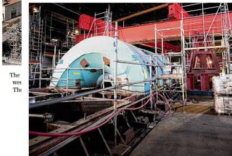
Workers replaced the Unit 8 generator after the previous one was destroyed by a fire last year.
