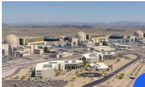
Palo Verde Nuclear 3,940 MW Arizona
